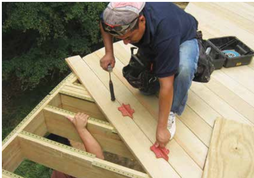
Figure 1. When wood decking is installed, the gaps between the deck boards should be sized according to their moisture content at the time of installation. Kiln-dried decking will require wider gaps than wet lumber.
