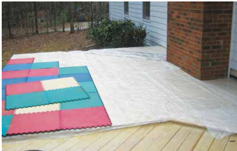
Figure 6. After installation, the author protects wood decking from rain and construction damage with a layer of plastic. The interlocking rubber mats provide additional impact protection and limit UV exposure.
