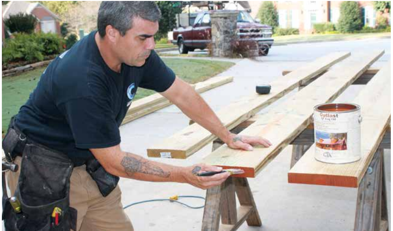
Figure 2. End cuts and bolt holes in pressure-treated decking and framing should always be re-treated with a wood preservative prior to installation. Sealing the ends of the boards with a penetrating oil will help block moisture absorption through the end grain, which will limit cracking and checking.
